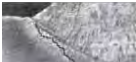
Welding Inspection: Crack through HAZ
