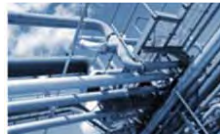
New Construction Surveillance
