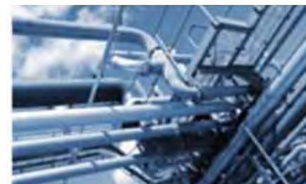
New Construction Surveillance
